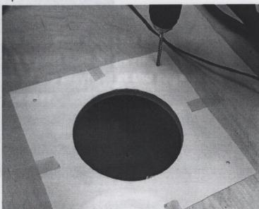
23) If the cabinet is a bit rough from the chisel, use a sanding block to smooth it down. This will be covered by the new speaker and not visible.
