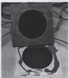
21) Use the included template to mark the four holes for the new woofer. Align the center hole in the template so it is concentric with the hole in the speaker floor and parallel to the sides of the cabinet; then tape the template in place. 22) Use the included drill bit to make the four pilot holes for the screws, and then remove the template. Drill the pilot hole ¼" deep. You can also make some marks on the bottom of the playfield at the edge of the template to help you align the new speaker.
